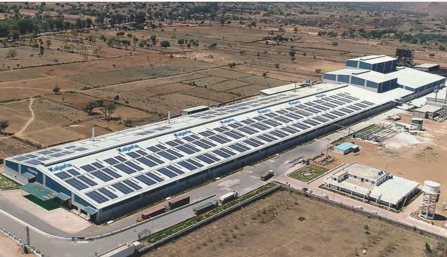
Aerial view of Virat Nagar Plant (Rajasthan)
